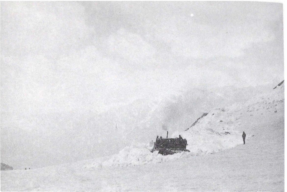
3. The road is being cleared with the help of bulldozer.
