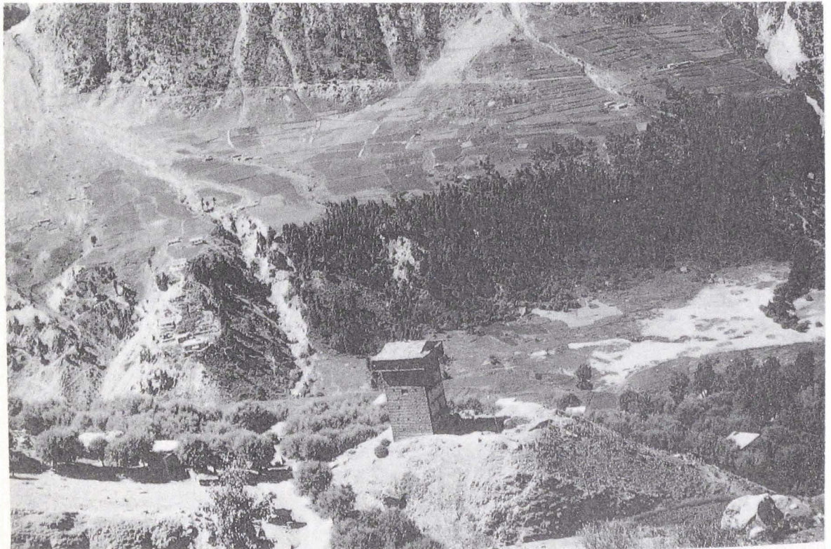
12. The Fort of Gondhla.
